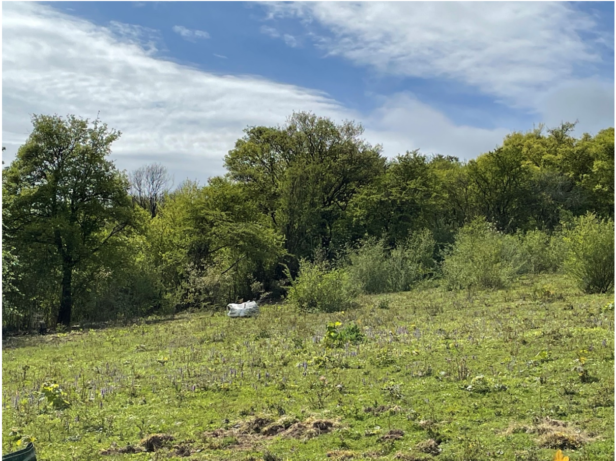
Image of work commenced within field (left side completed/right side not completed)
