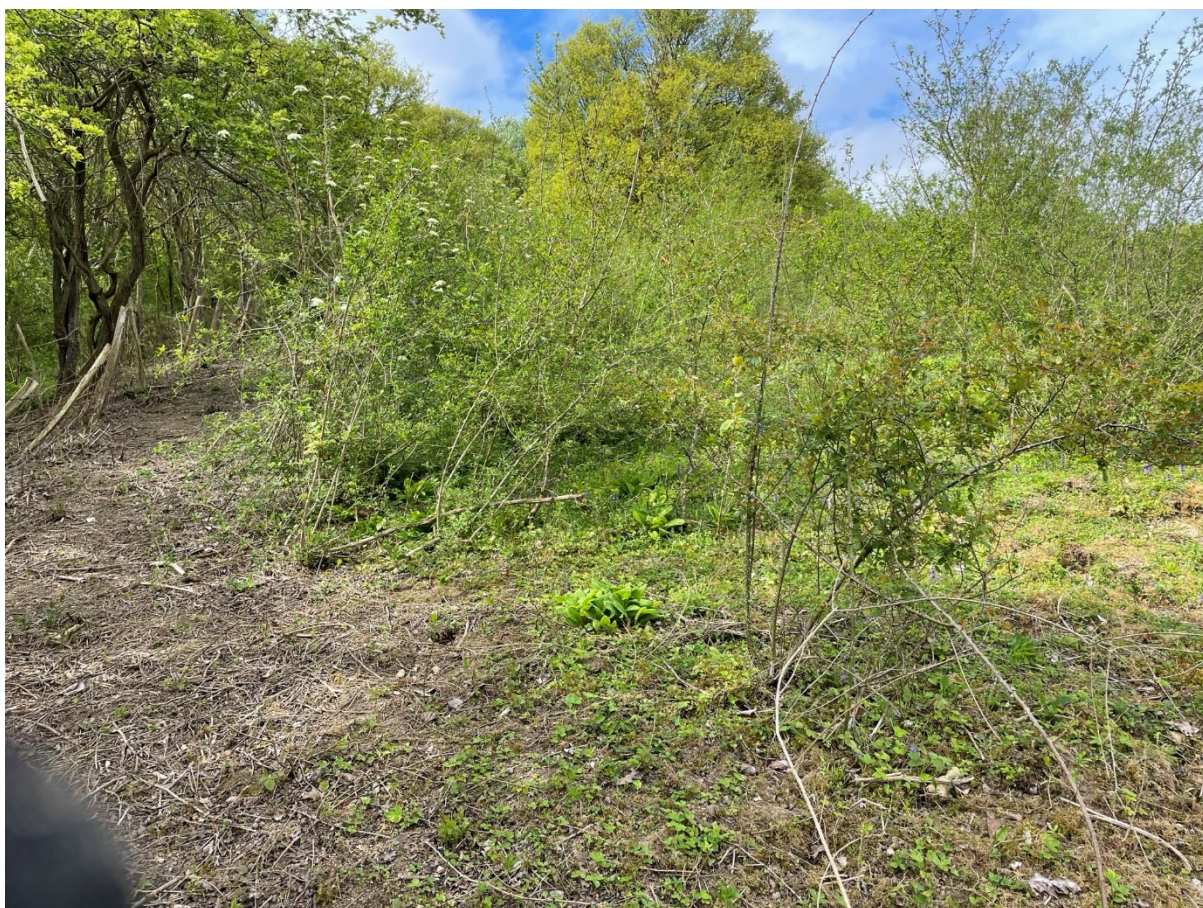
Boundary being cleared to enable the boundary fence to be repaired.
