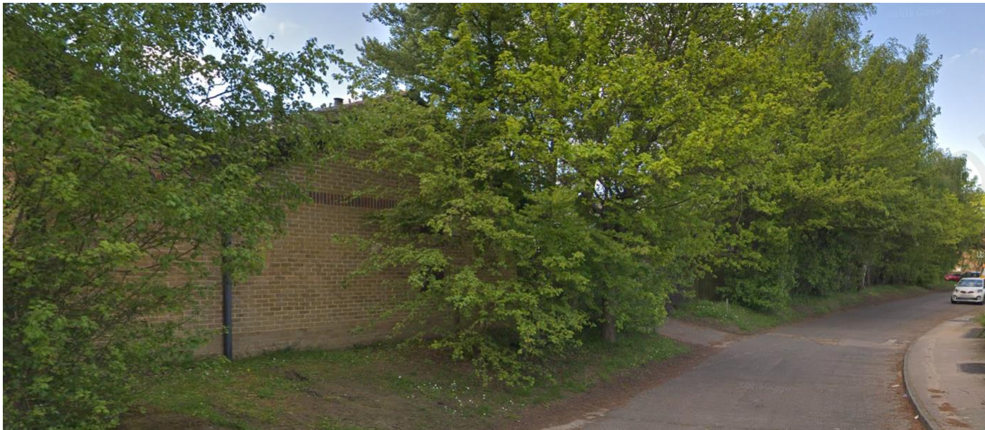
Plate 12: View of the rear of the PDA (facing SW).
