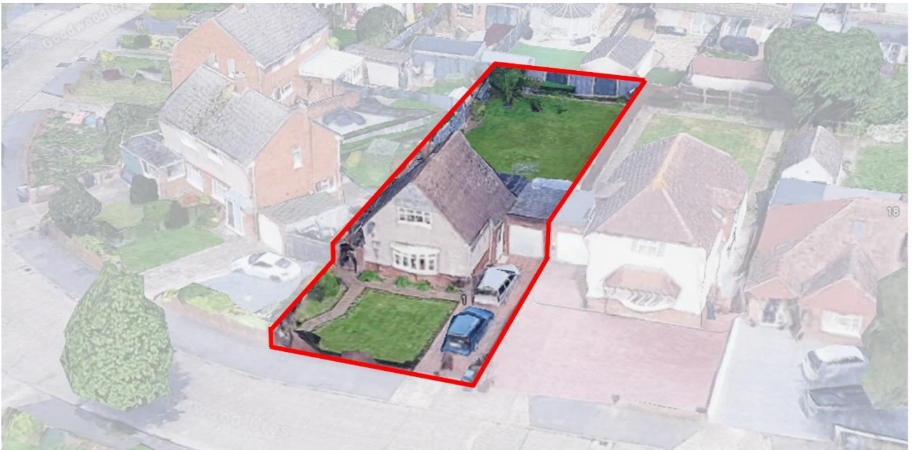
No. 22 Goodwood Crescent, Gravesend, Kent DA12 5EL Existing Aerial View
