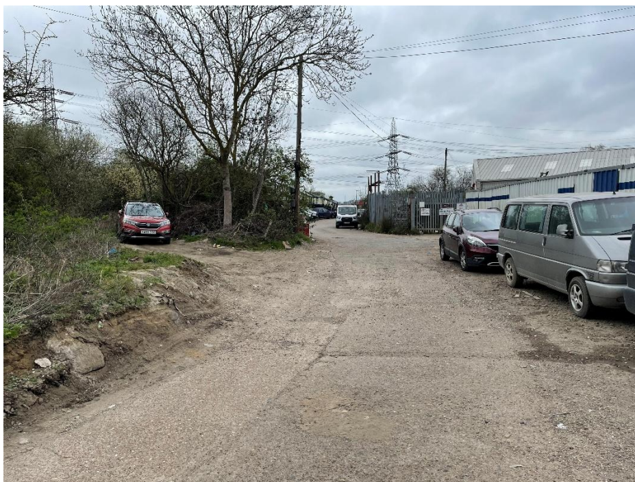
Photograph 2.5 – Example of verge overrun along Queens Farm Road close to the junction with the business park service road
