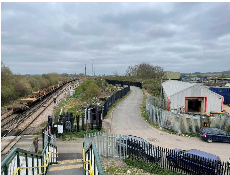
Photograph 2.10 – The North Kent Line Main to the left and Apex Business Park to the right
