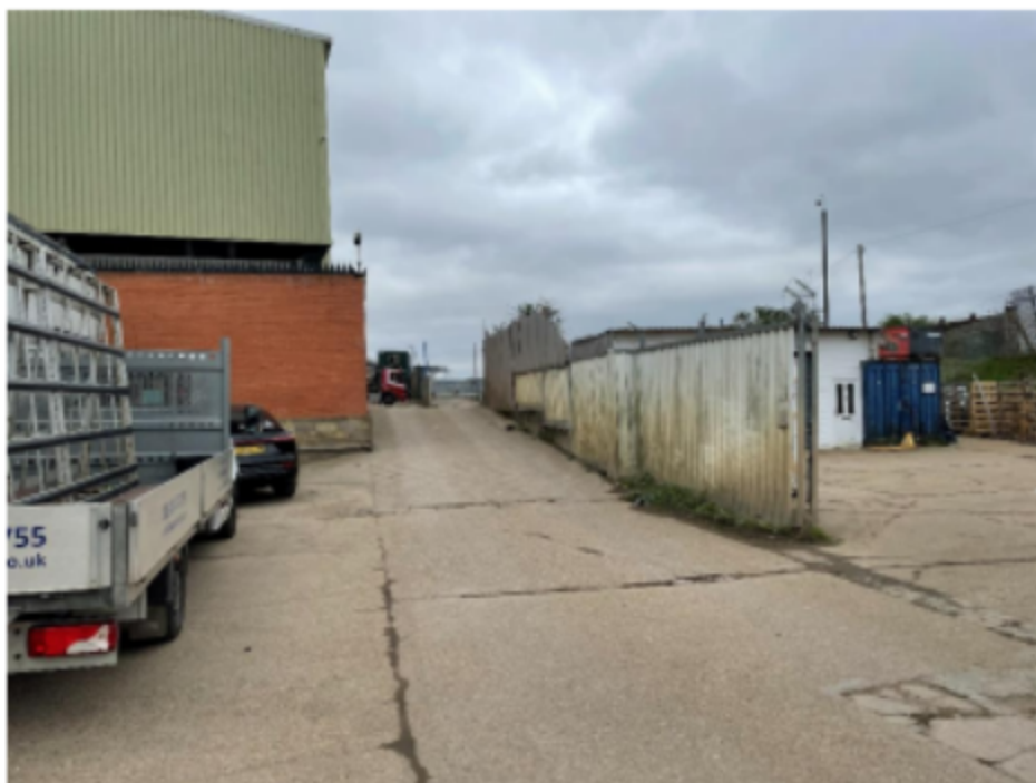
Photograph 2.8 – The business park service roads narrows to a pinch point of 4m in width at around its midpoint but good intervisibility is maintained
