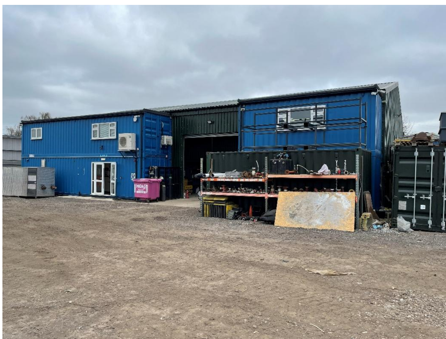
Photograph 3.1 – The temporary structure
