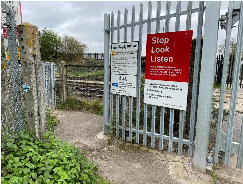
Photograph 2.12 – At grade crossing of the North Kent Line
