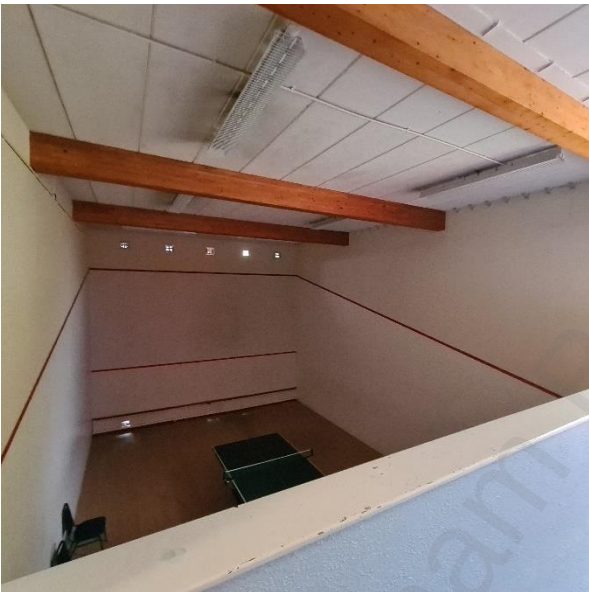
Figure 30: Exposed roof structure above squash courts 3 to 6
