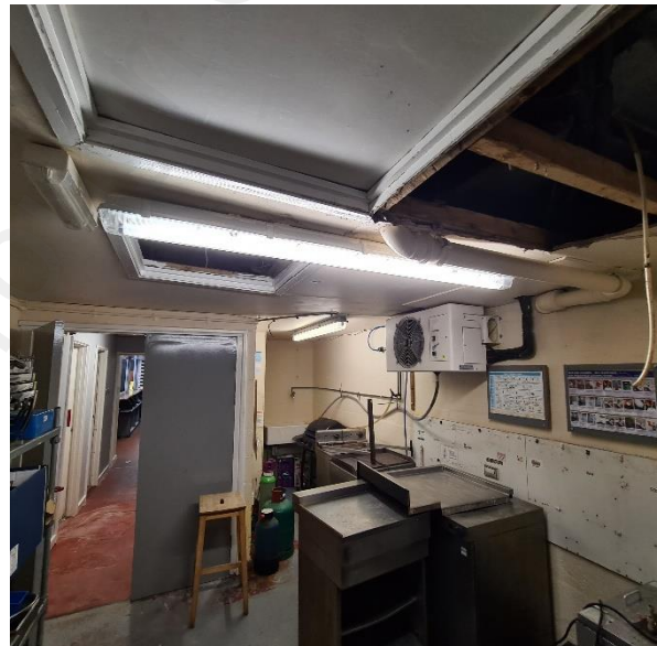
Figure 67: Ground floor store room
