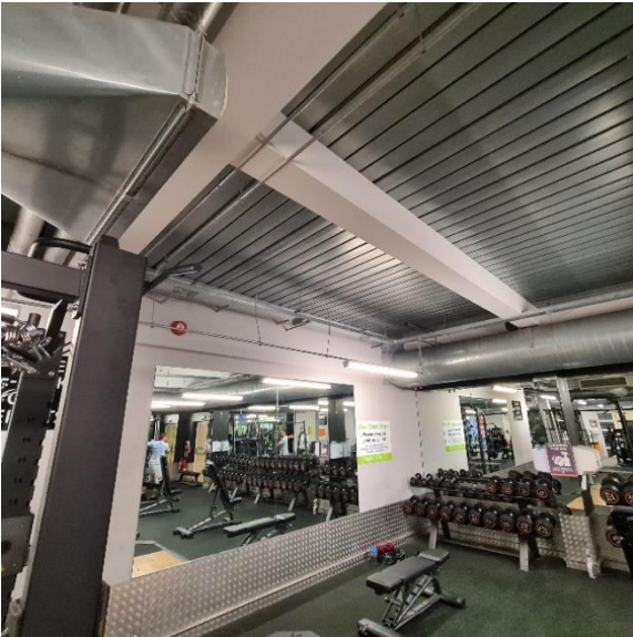
Figure 40: First floor exposed structure soffit
