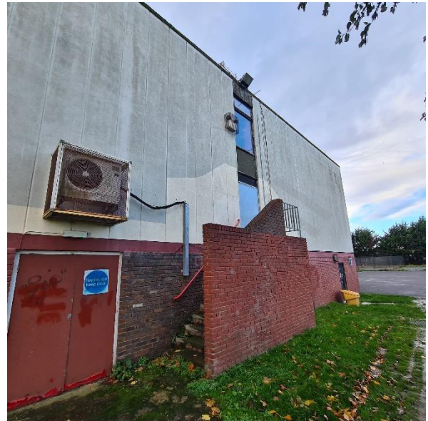
Figure 76: North elevation of squash courts
