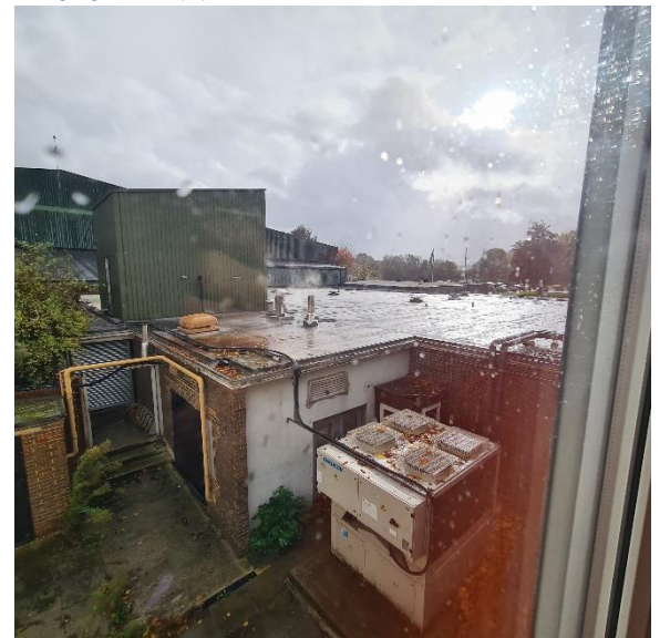
Figure 21: Flat roof over original building area
