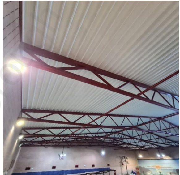
Figure 43: Pool hall exposed roof structure (3)
