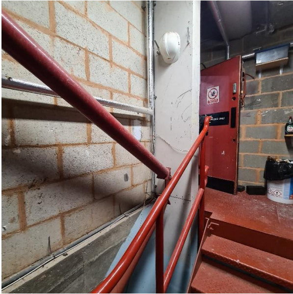
Figure 52: Pool plant room exposed structure
