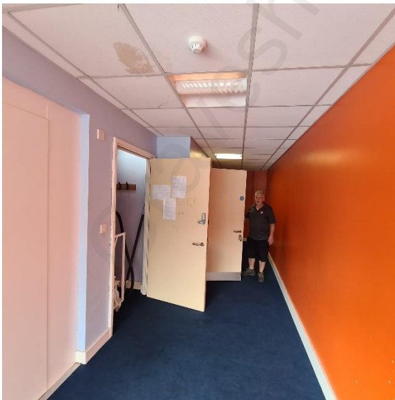
Figure 26: Cupboards adjacent to courts 1 & 2
