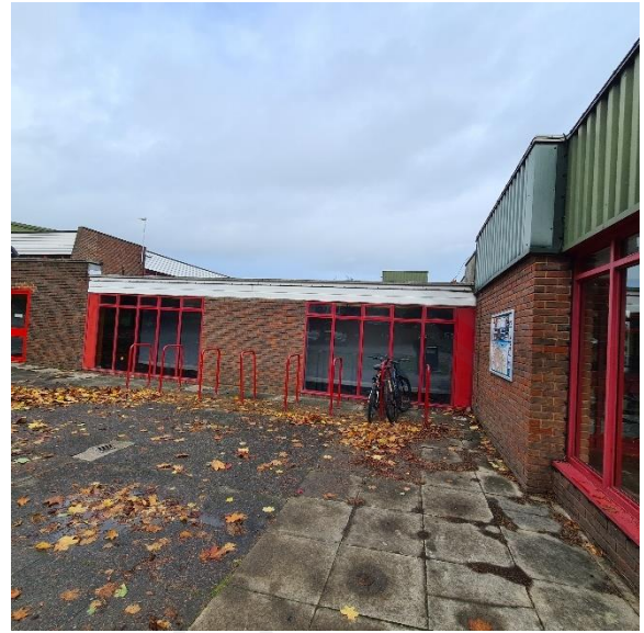
Figure 70: South elevation of original building
