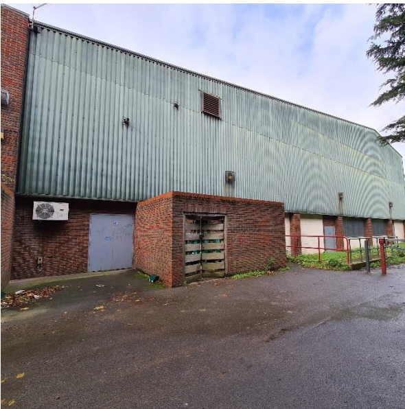
Figure 83: East elevation of pool hall
