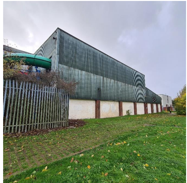
Figure 82: North elevation of pool hall
