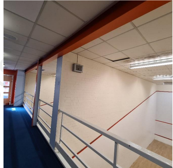
Figure 25: Structural steel framing adjacent to courts 1 & 2
