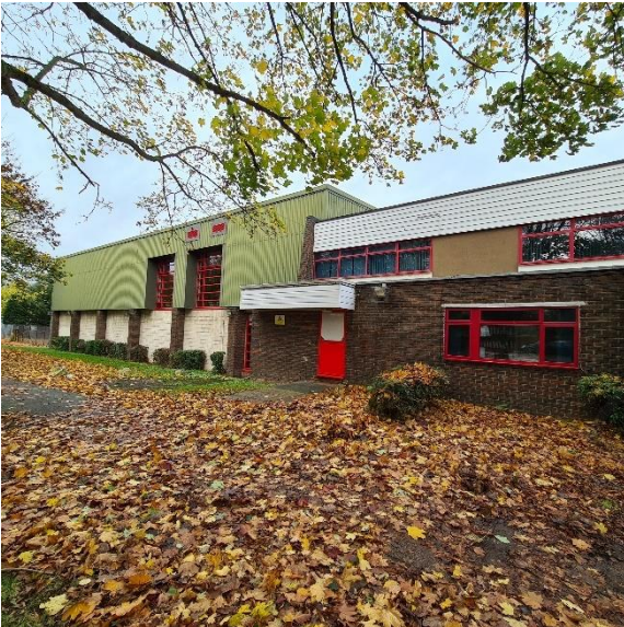
Figure 71: South elevation of original building and sports hall
