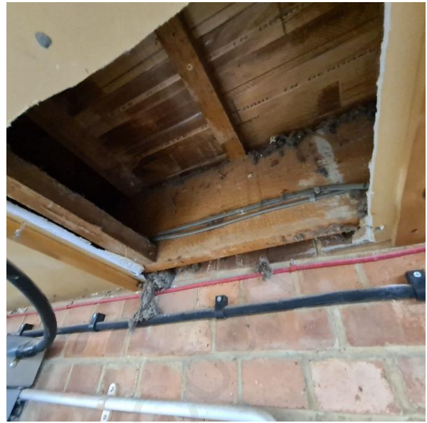
Figure 29: Suspended ground floor construction to squash courts 1 & 2
