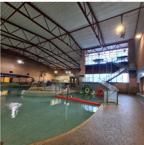
Figure 44: Pool hall exposed roof structure (4)
