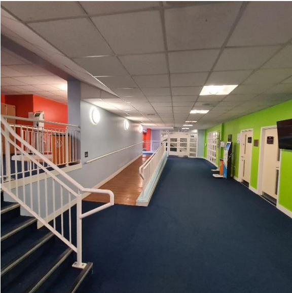
Figure 22: Stepped and ramped access down to lower ground level of original building
