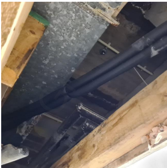
Figure 68: Exposed first floor structure soffit
