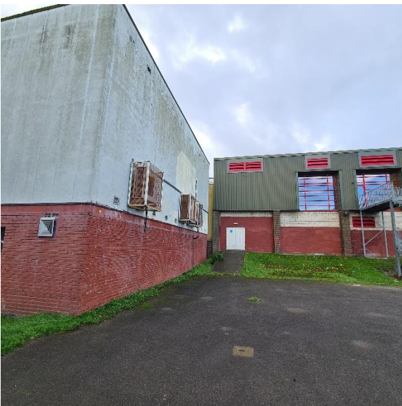
Figure 77: West elevation of squash courts
