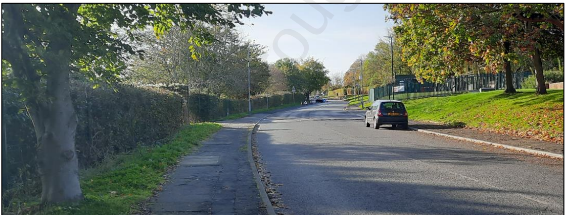
View looking south on Thong Lane showing footways on both sides
