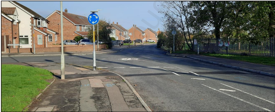
View looking north on Thong Lane towards junction with Leander Drive
