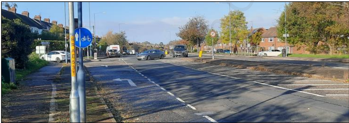
View looking west on A226 towards junction with Thong Lane
