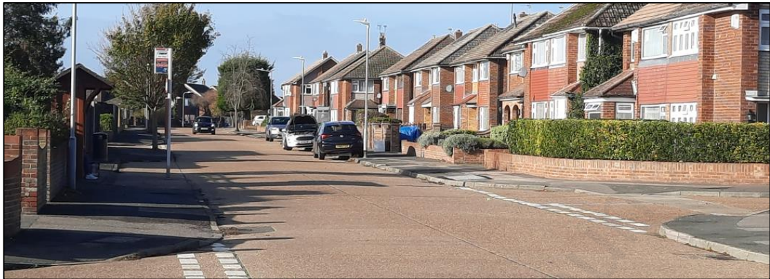
View looking west on Vigilant Way
