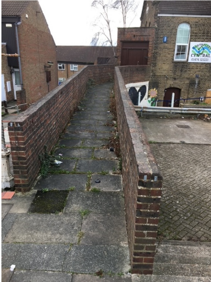
Fig vii: View of ramp to first floor.
