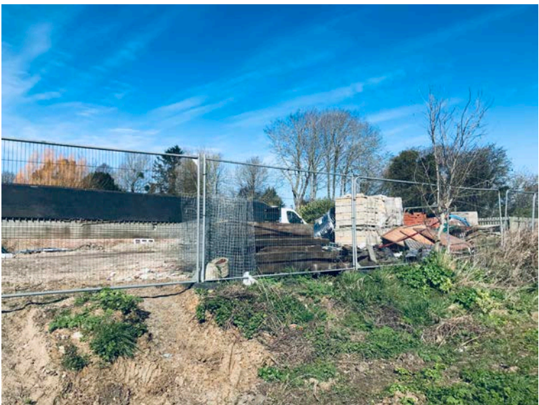
Construction storage on made ground in the storage yard.
