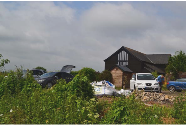
Cobhambury Barn, now residential, marks the eastern edge of the farm cluster whilst parking and storage occupies land to the east.
