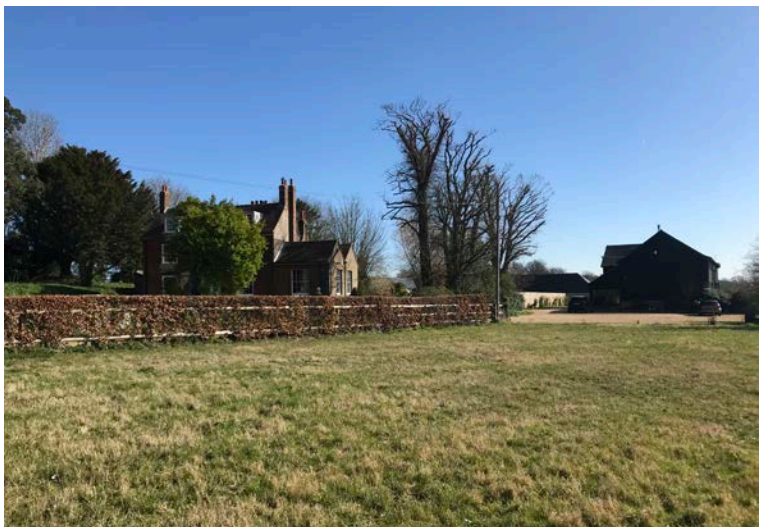
The hierarchy of buildings; farmhouse to the left, Cobhambury Barn to the right, and behind the trees, the single storey animal building now workshops, accommodation and offices. The oast which would have been in the foreground, completing the group, is now absent.
