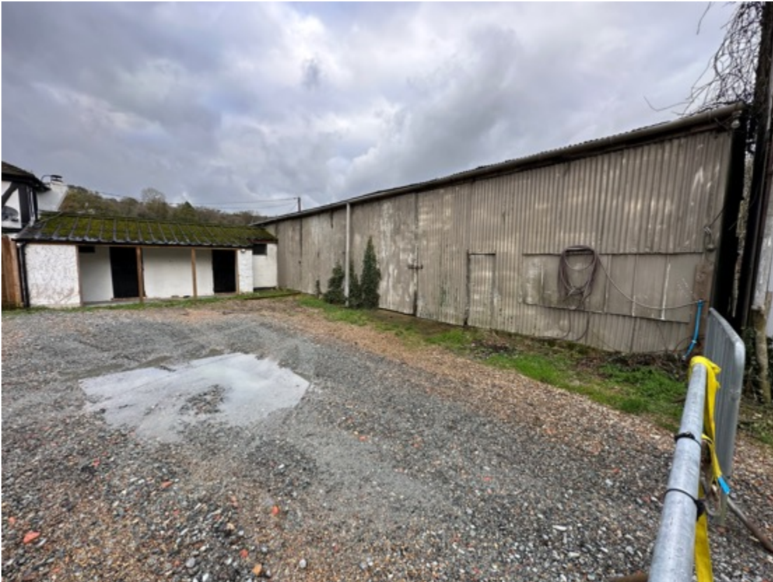
Photograph 5: Southern aspect - stables and western aspect - northern agricultural building
