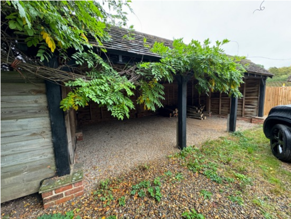
Photograph 11: Front of the car port, looking north-west – surveyed for bats, none present
