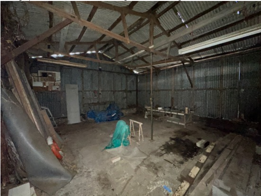
Photograph 8: Interior of the northern agricultural building
