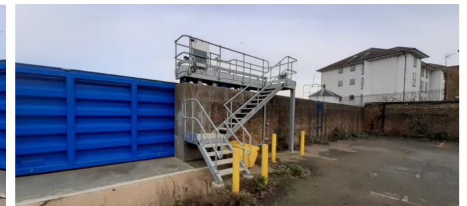
Photograph of Flood defence wall, flood gate and existing staircase.
