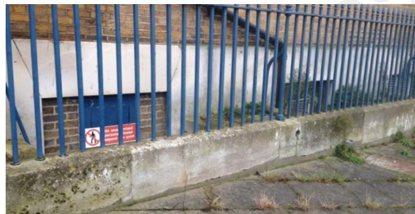
Photo of side elevation light wells
