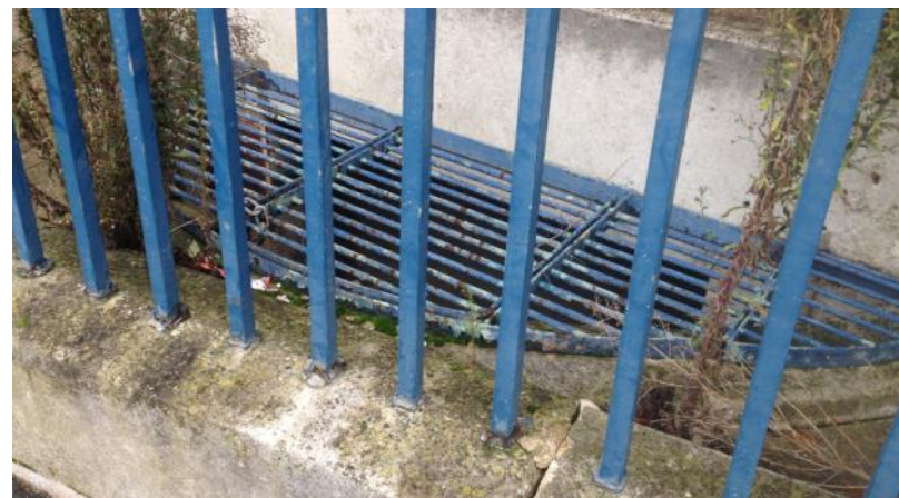
Photo of front elevation light well
