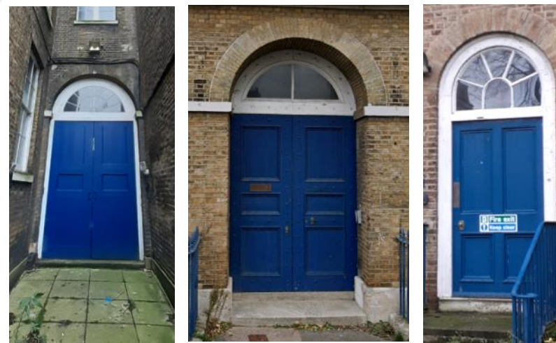
External doors to be refurbished and retained.
