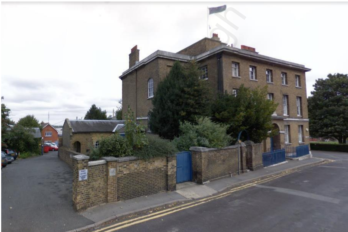
Fig 27 The Custom House in 2008 in its latter years as HM Customs & Excise offices with the agency's flag flying from the flagpole, showing the unkempt yards at the front and the extensive use of the north yard for parking.
