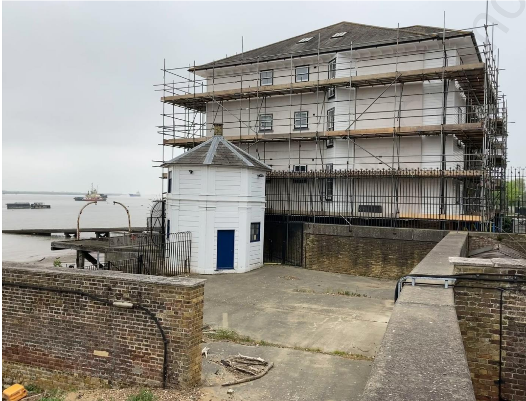
Fig 62 The Gazebo outside the flood wall with the yard around it and potential access from Heritage Quay
