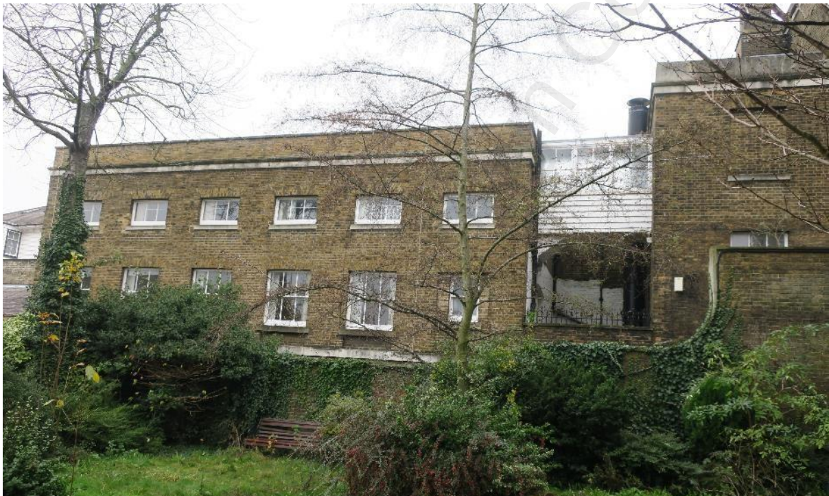
Fig 45 view of the first range of the outbuildings range running down to the river
