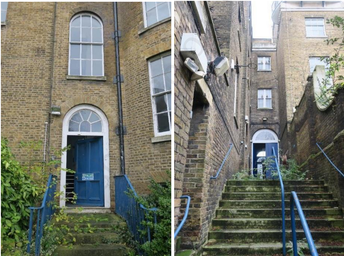
Figs 30 & 31 The entrance to the main staircase in the centre of the north elevation and the passage to the street entrance
