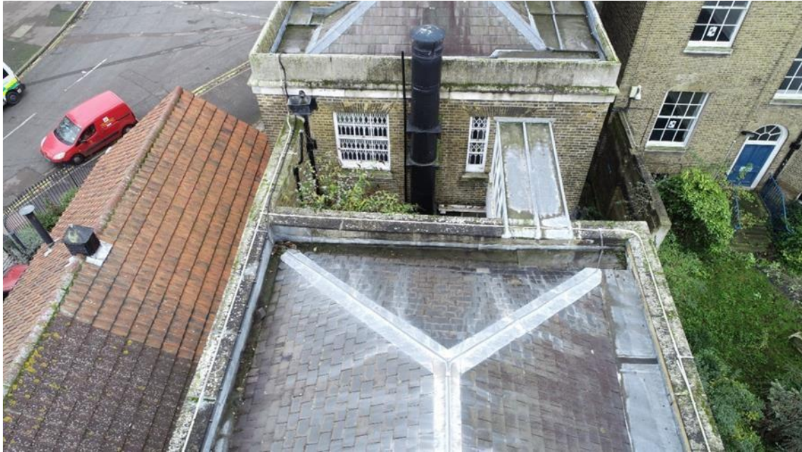
Fig 56 View of the lower bay on the north of the east wing showing where the early 20 th century bridge is attached awkwardly taking out 2/3 of the original sash window, though the rubbed brick arch over remains.
