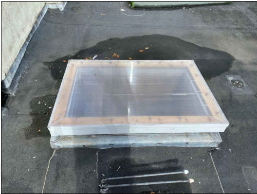
Existing polycarbonate rooflight RL01 - External view 1
