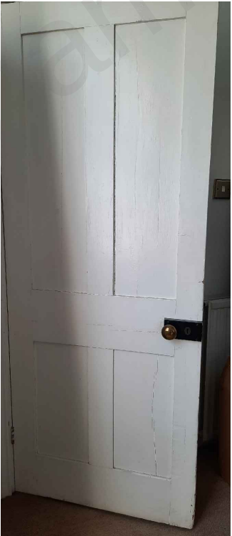
Typical existing internal timber door
