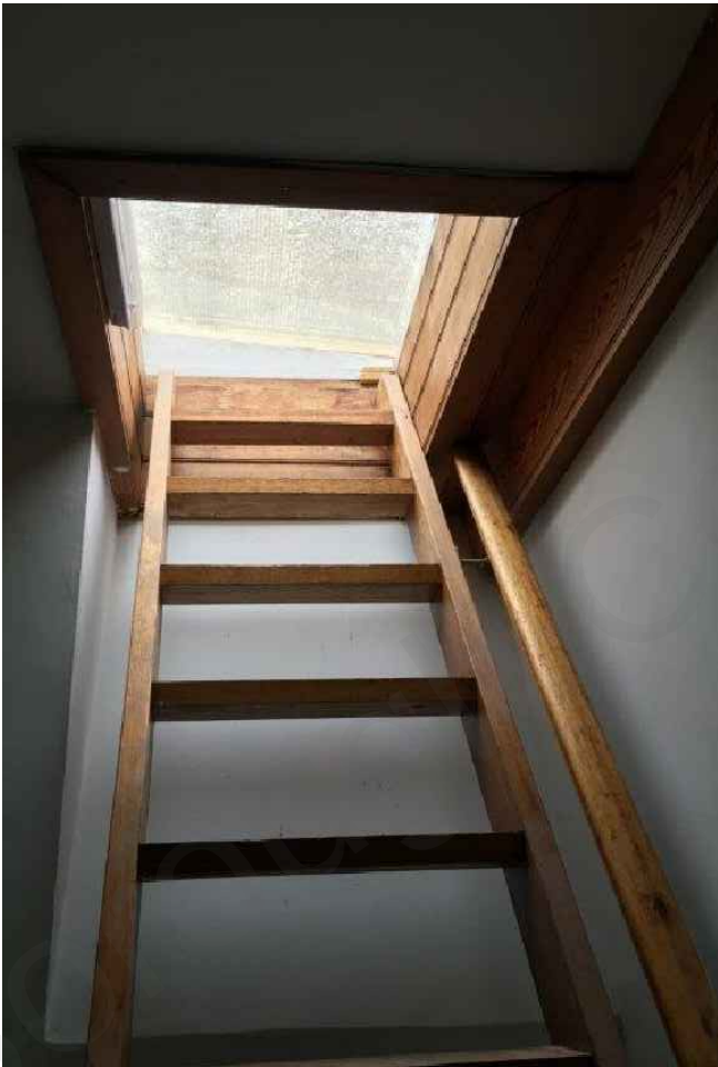
Existing polycarbonate rooflight RL01 - Internal View
