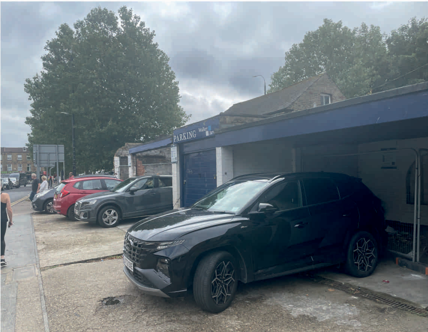
EXTERIOR - Lord Street existing parking forecourt
