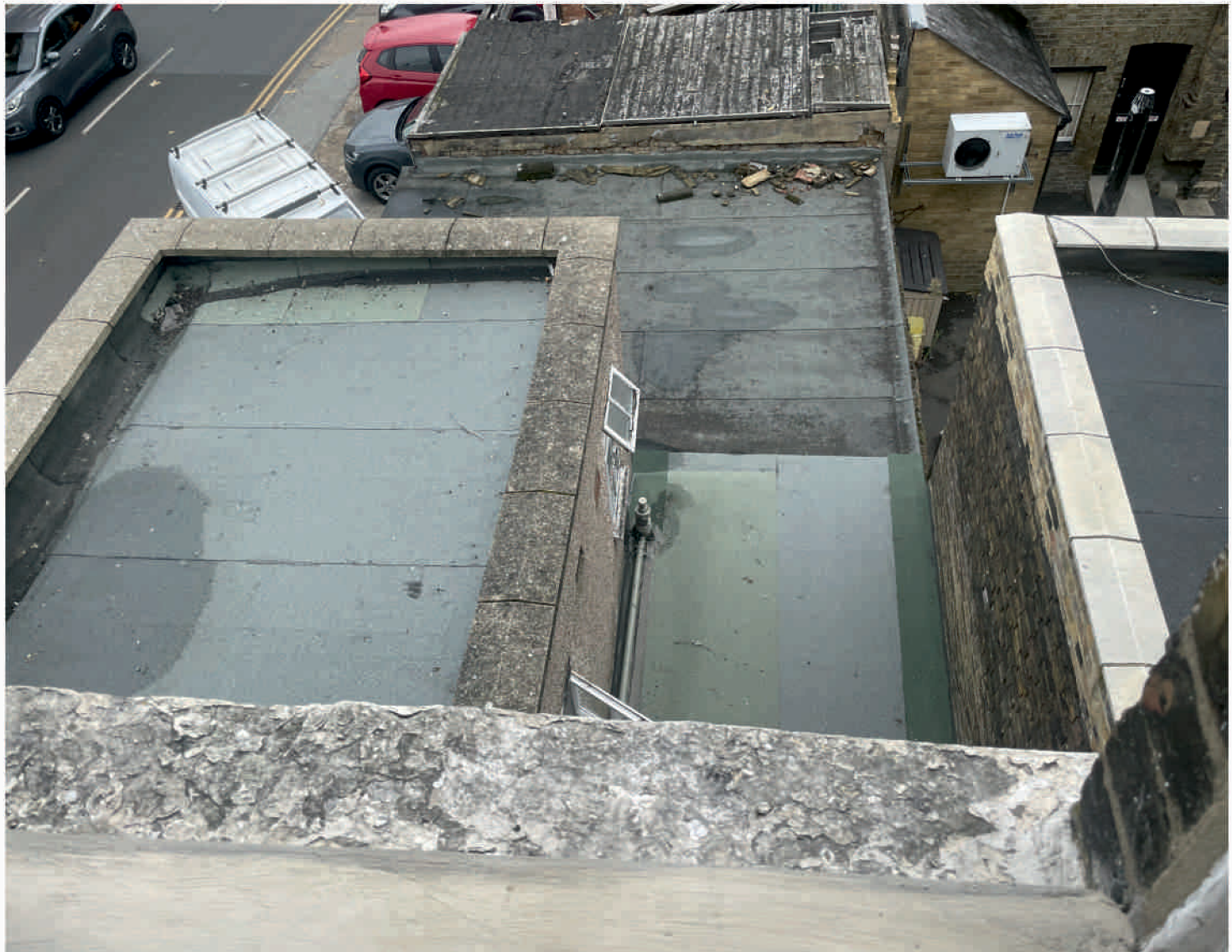
EXTERIOR - L-view of roofs to the rear from the window of room 19
