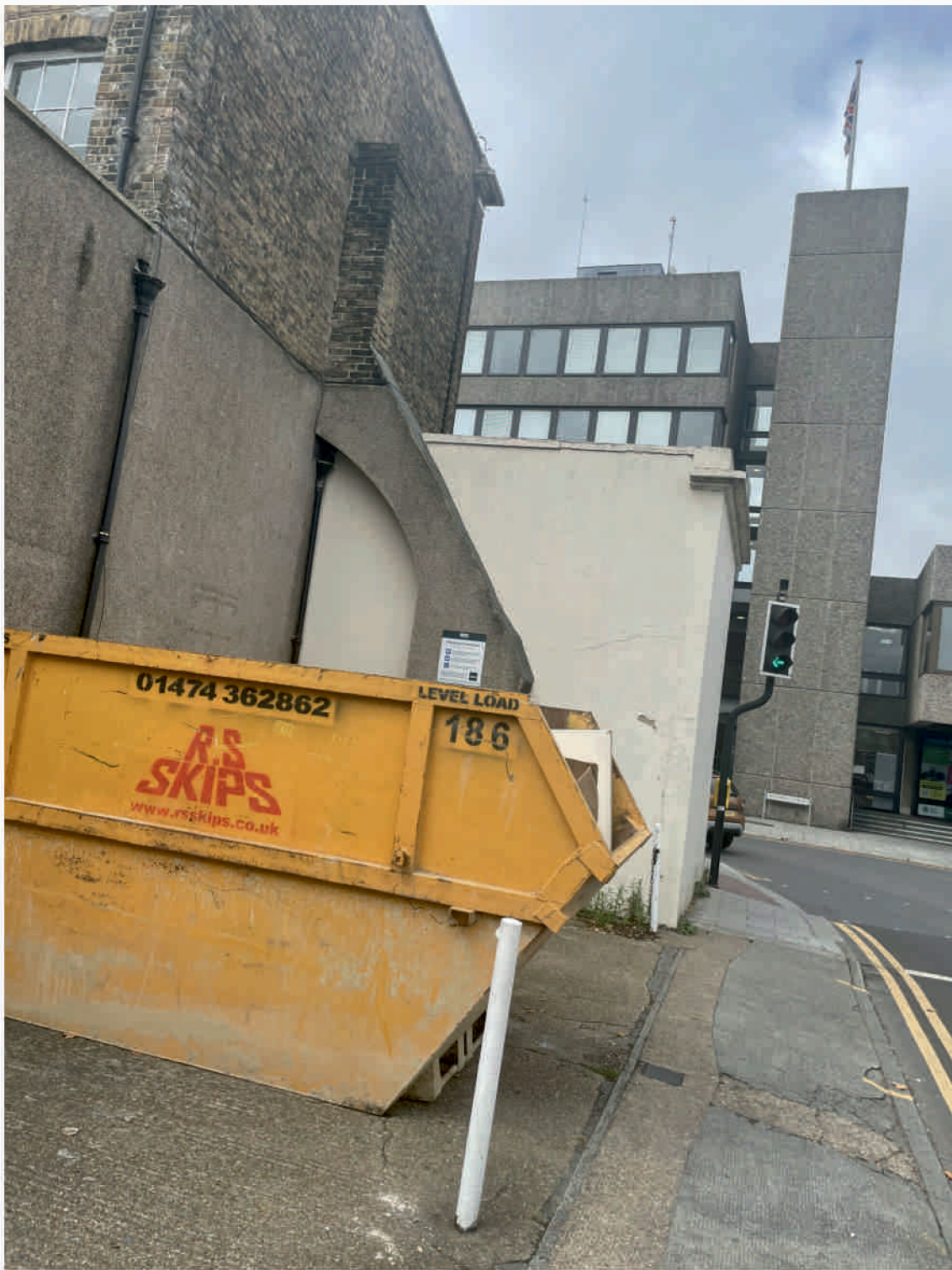
EXTERIOR - Rear of single storey element to the side
