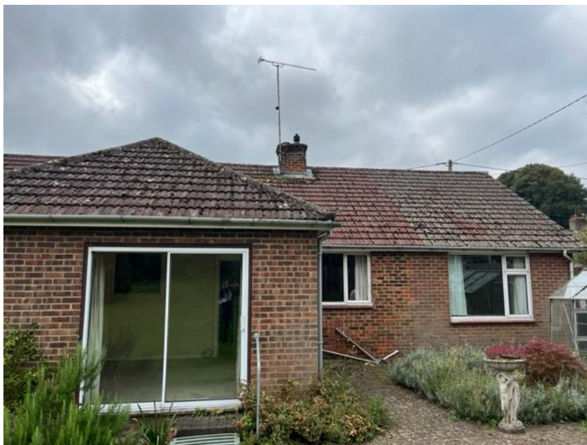
View of the side and rear extensions
