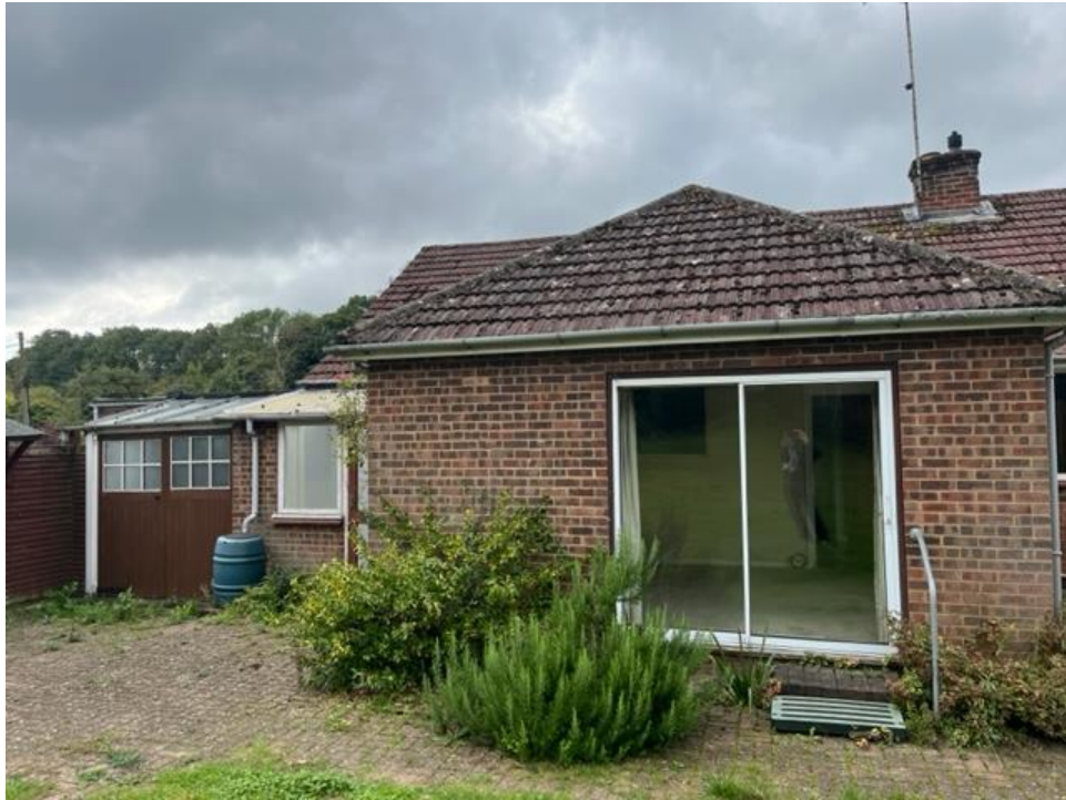
View of the rear extensions to original house
