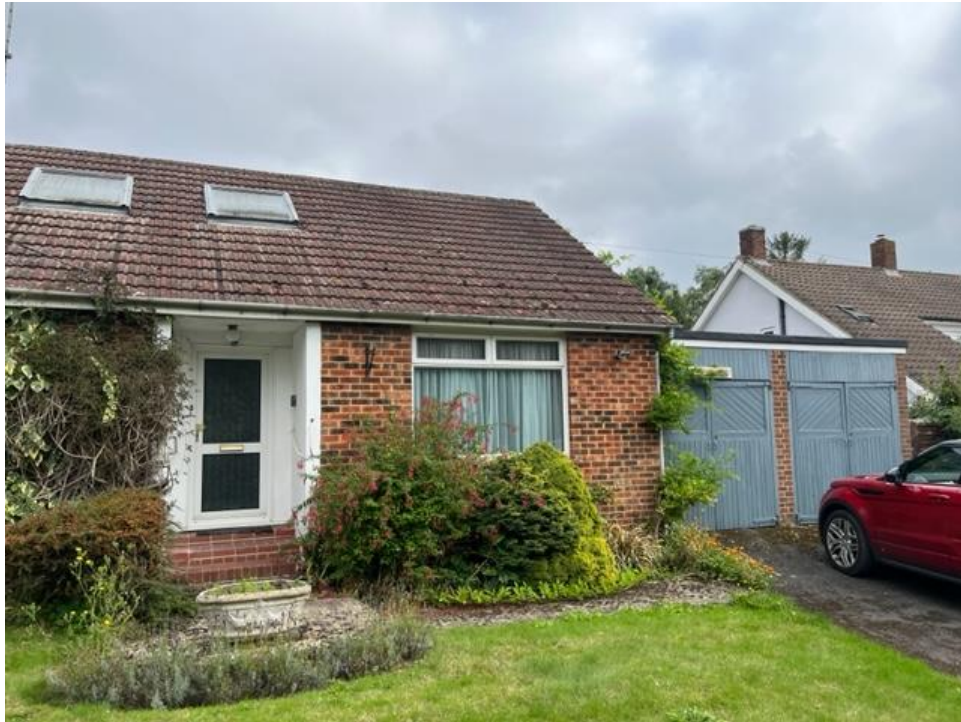
View of front of house showing poor quality linked double garage and driveway
