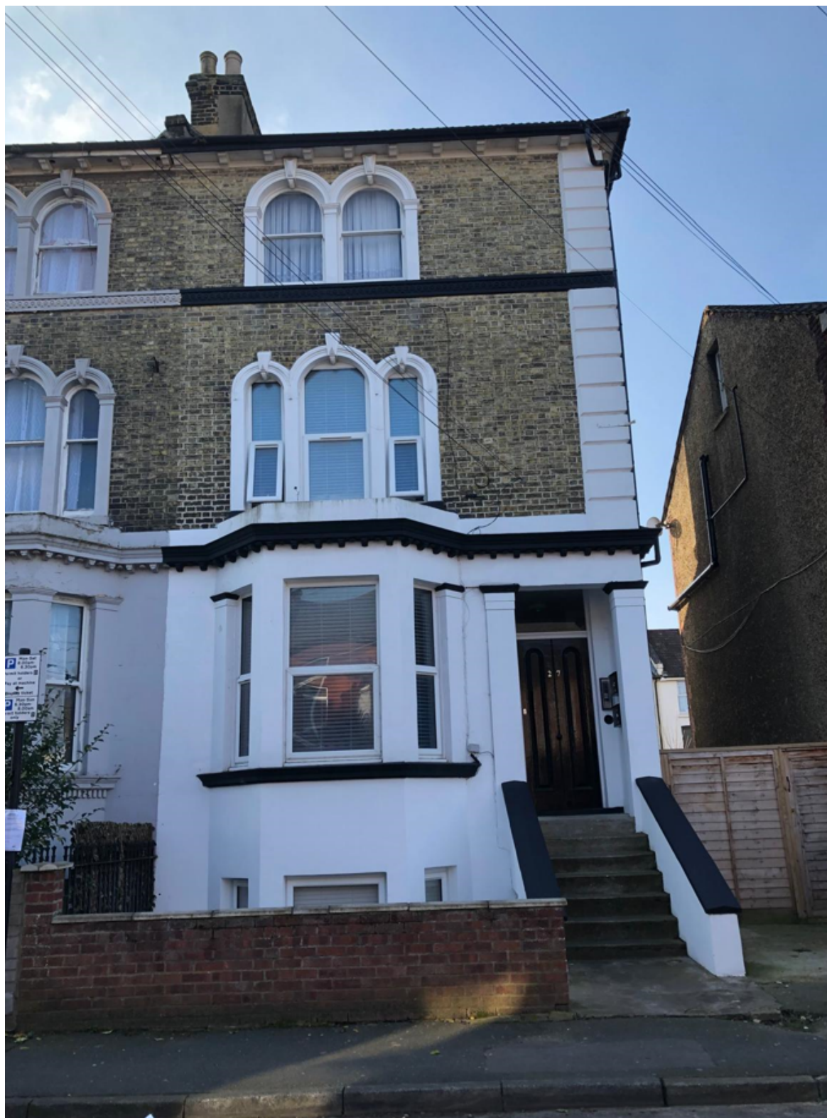
Site photo February 2025
