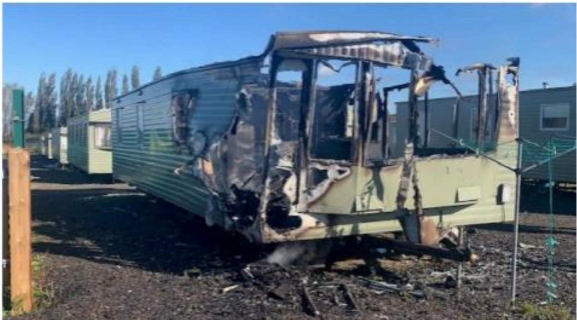
Figure 4 Photo showing worker's accommodation that was damaged by a fire.
