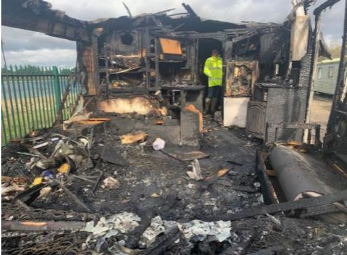
Figure 5 Photo showing worker's accommodation that was damaged by a fire.
