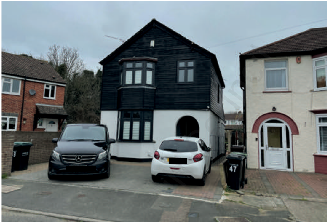
49 Gouge Avenue front view | existing 3-bedroom detached dwelling
