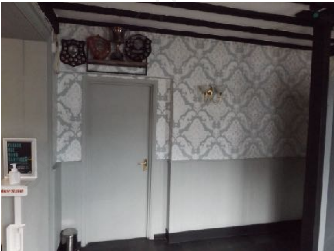
Recessed partition to be removed
