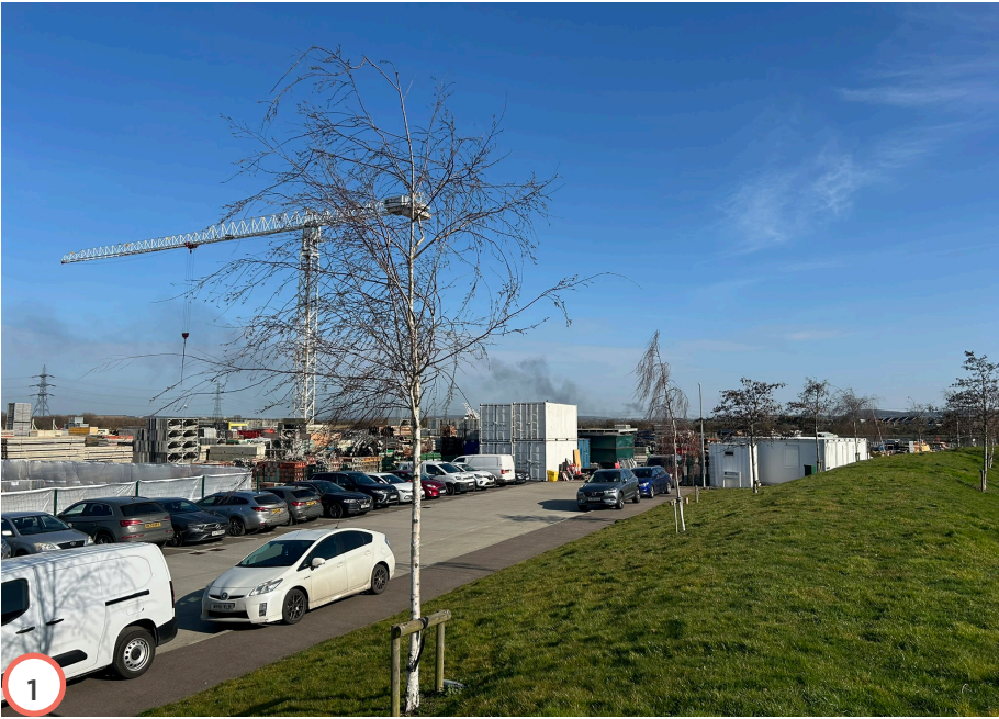
From the neighboring industrial yard, the site has a low profile with a flat topography and backdrop. There is currently nothing protruding the skyline.
