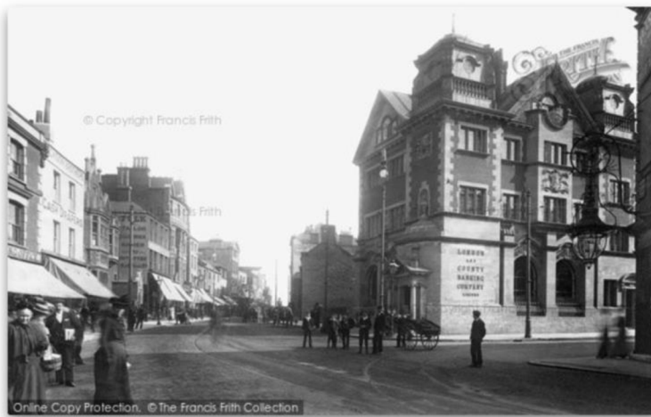
Gravesend, King Street 1902 Photo ref: 49028
