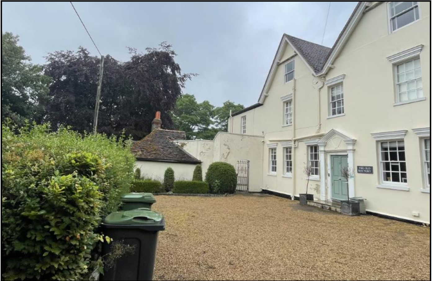
Image taken during the site visit
