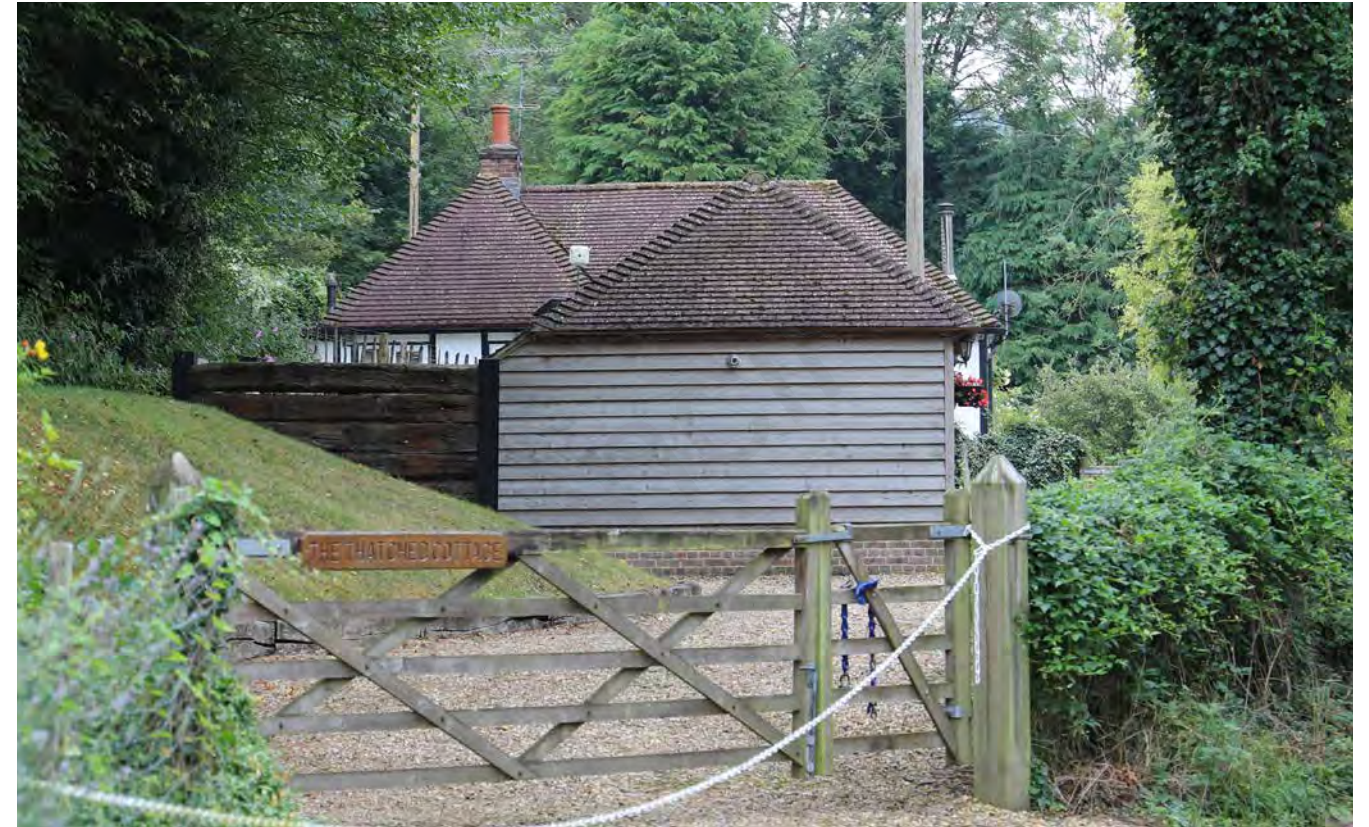
Tile roof, pitched roof, brick chimney, timber clad car port
