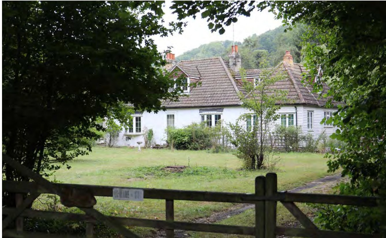
Tile roof, Dormer bungalow style, brick chimneys, white painted brickwork, PVC windows
