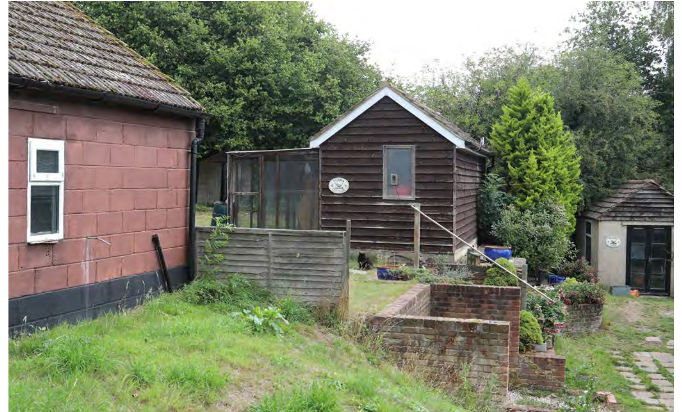
Pitched roof, coloured breeze block walling, timber cladding, PVC windows
