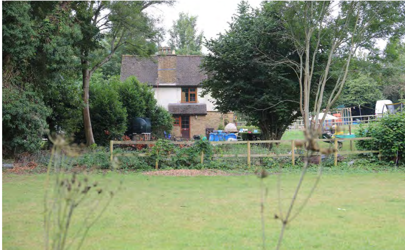
Pitched roof, brick chimneys, timber window frames, rendered brickwork walls
