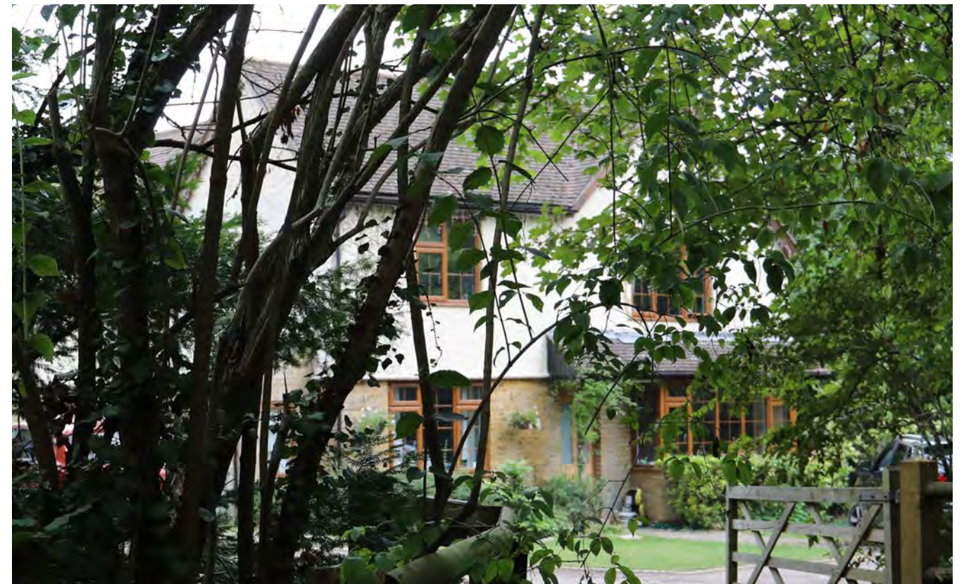
Pitched tile roof with brick chimneys, white painted brickwork, timber window surrounds, lower facing brickwork
