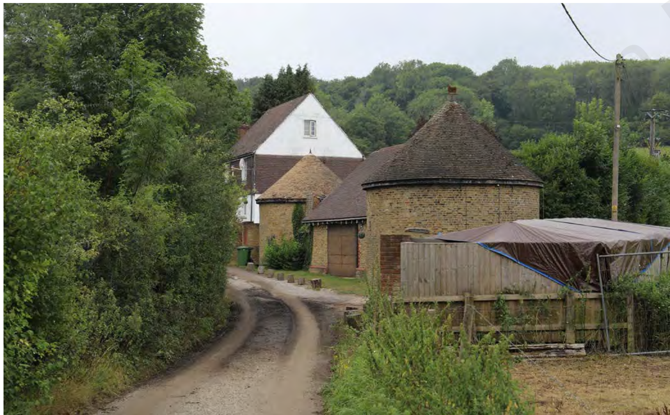
Tile roof, brickwork building, white painted brickwork, pitched roof
