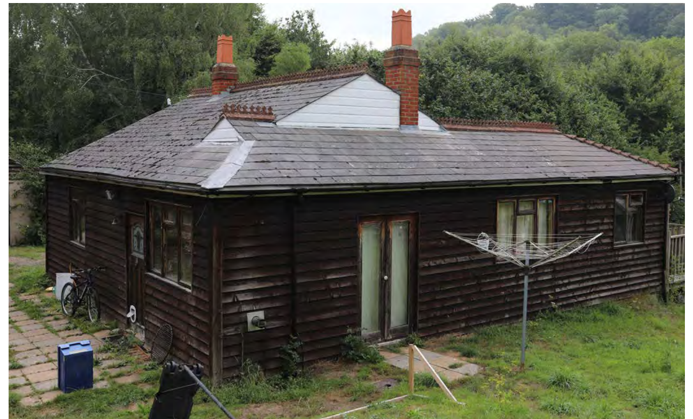
Timber cladding, slate roof, pitched roof, white painted brickwork, brick chimneys
